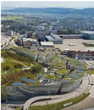
The Circle – airport, Zurich, Switzerland
